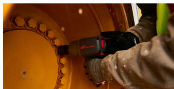
Heavy Equipment Repair
